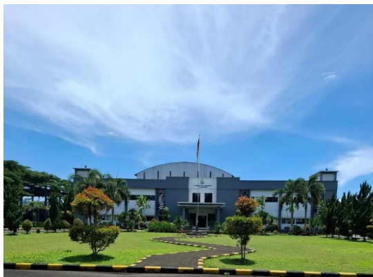
Gambar 1 PT Sinergi Gula Nusantara Unit Pabrik Gula Glenmore
